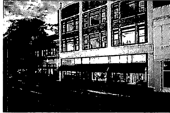
Corporate Headquarters, Sumter, SC
